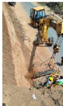
Soil nailing work being undertaken by the State Highways Department in the Nilgiris. SPECIAL ARRANGEMENT
