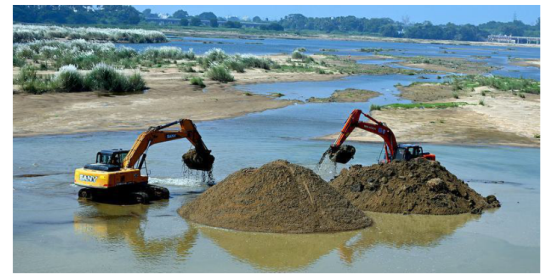
Initial stage: A view of the bund created around a test pile foundation on Cauvery river for the new bridge at Tiruchi on Wednesday. M. MOORTHY
