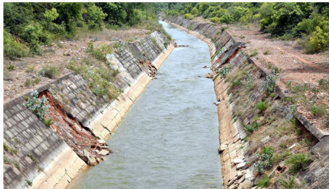
Reducing seepage: Damaged portions of the Kandaleru-Poondi Canal will be strengthened with a slope protection lining and retaining wall for nearly 2 km at a cost of ₹10.20 crore. FILE PHOTO
